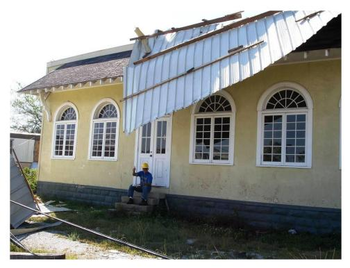
Figure 7-5 – Roof fragment falling hazard, 2005 Hurricane Katrina
