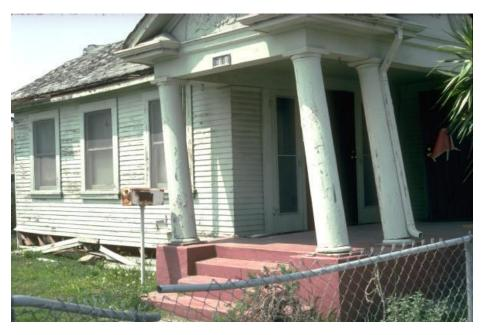
Figure 2-11 – Racking damage to porch, 1994 Northridge Earthquake
