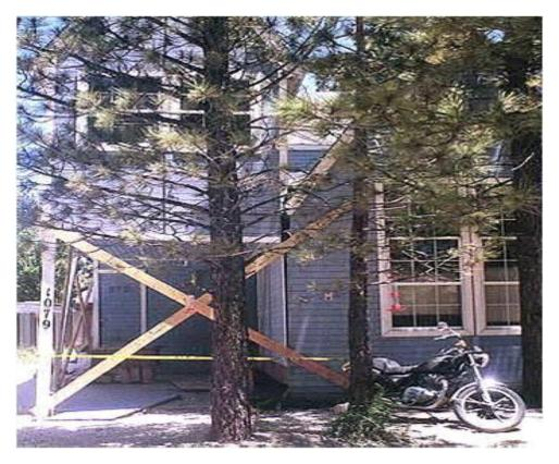
Figure 3-19 – Collapsed house with failing upper room, 1992 Big Bear Earthquake
