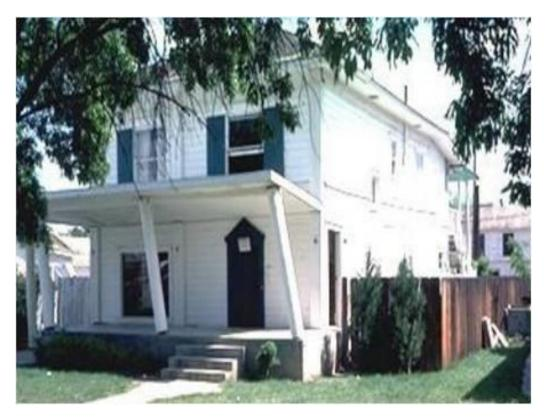
Figure 3-16 – House with cripple wall damage, 1983 Coalinga Earthquake
