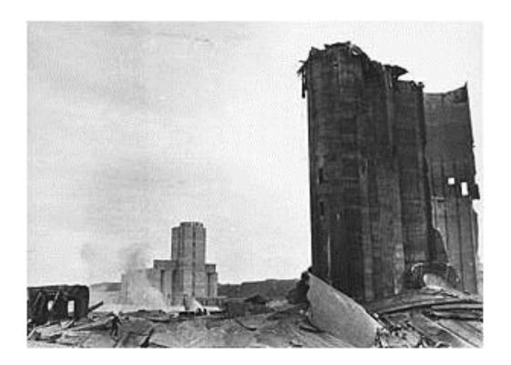
Figure 6-24 – Explosion – damaged granary
