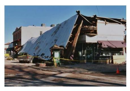
Figure 2-7 – Unreinforced masonry building with wall failure, 2003 San Simeon EQ
