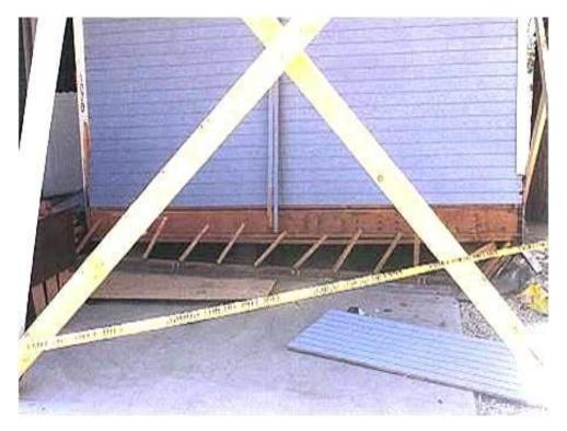
Figure 3-17 – House with cripple wall failure, 1992 Big Bear Earthquake
