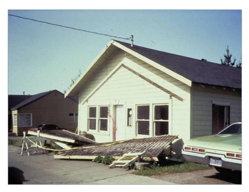
Figure 2-23 – Home with blocked front door, 1994 Northridge Earthquake
